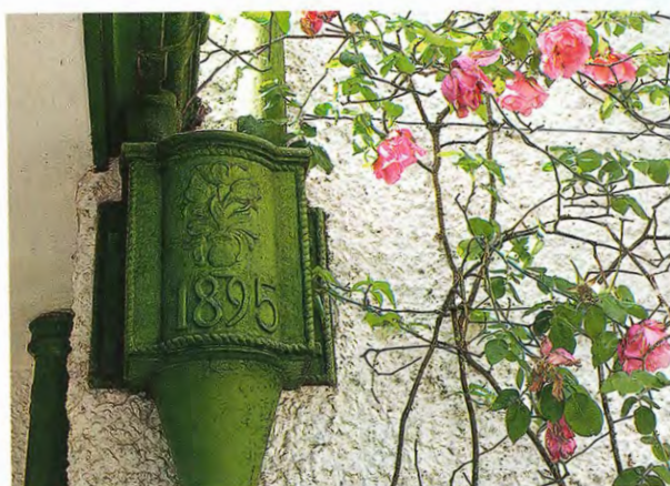
↑ Fig 5 left: Lily-decorated rainwater hopper.
